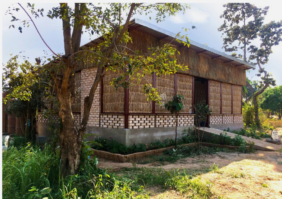
walls have been constructed using block made from local earth and other local resources including rice husks
