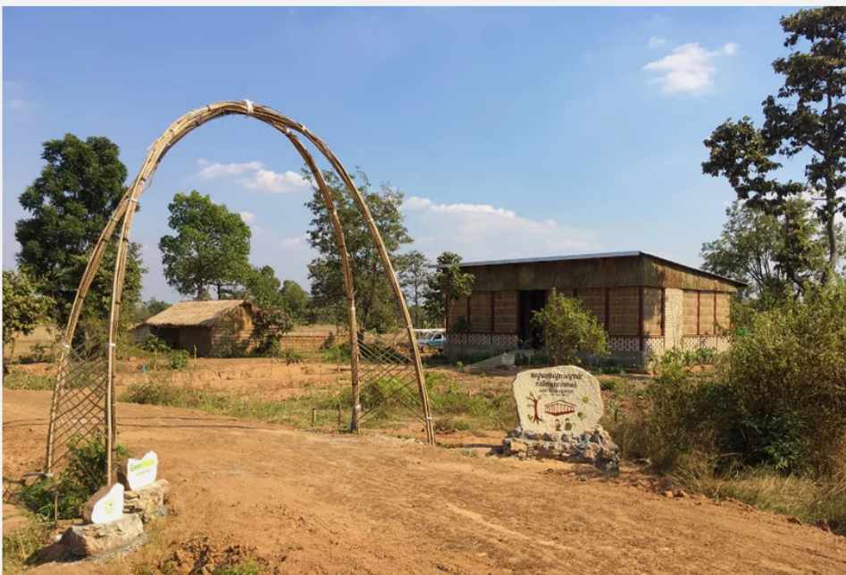
the robust steel frame is softened by using tactile local materials such as earth blocks and bamboo screens
