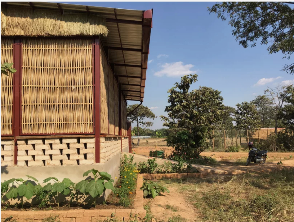
a wide roof canopy draws heavy rainfall away from the building edge
