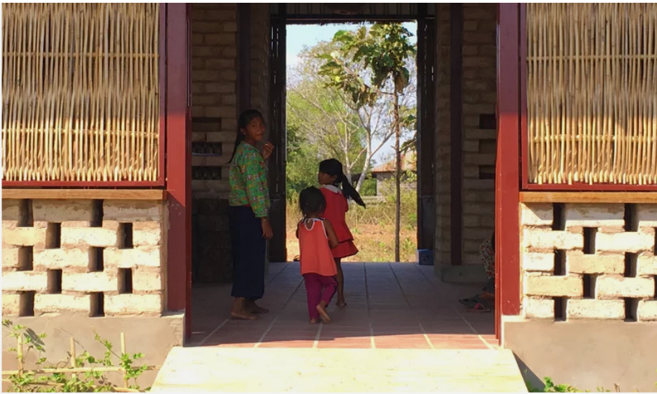
the entrance ramp leads through the social reception space into the classrooms to the rear
