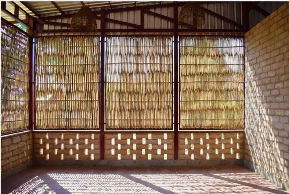
the robust steel frame is softened by using tactile local materials such as earth blocks and bamboo screens
